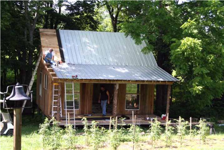
Putting on the roof
